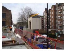
Lower Panels Positioned Over Standard Starter bars
